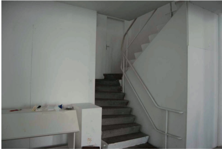
Halles USEGO inside view first floor
